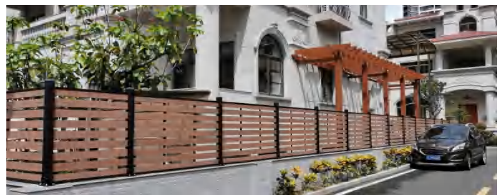
Jiangmen 1000meters Full-trellis Fence Project-2019
